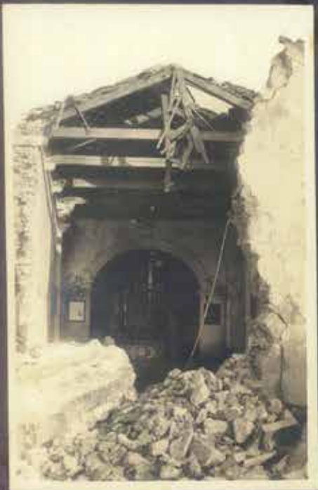
Remains of the old building after the earthquake
